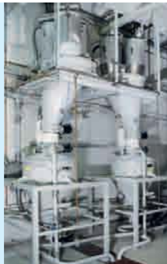
Central weighing station for long-lasting bakery products
