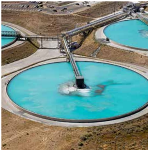
Sludge thickeners
